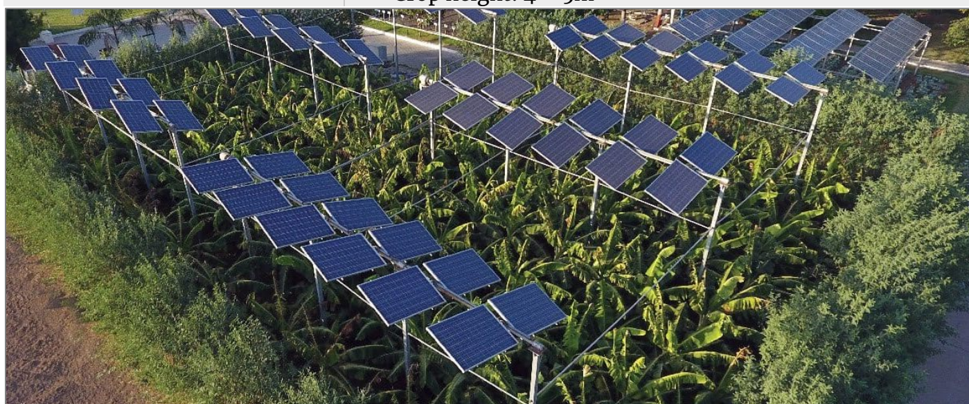
Figure 23: 14.4 kW agrivoltaic structure with banana (Credit: Jain Irrigation)
