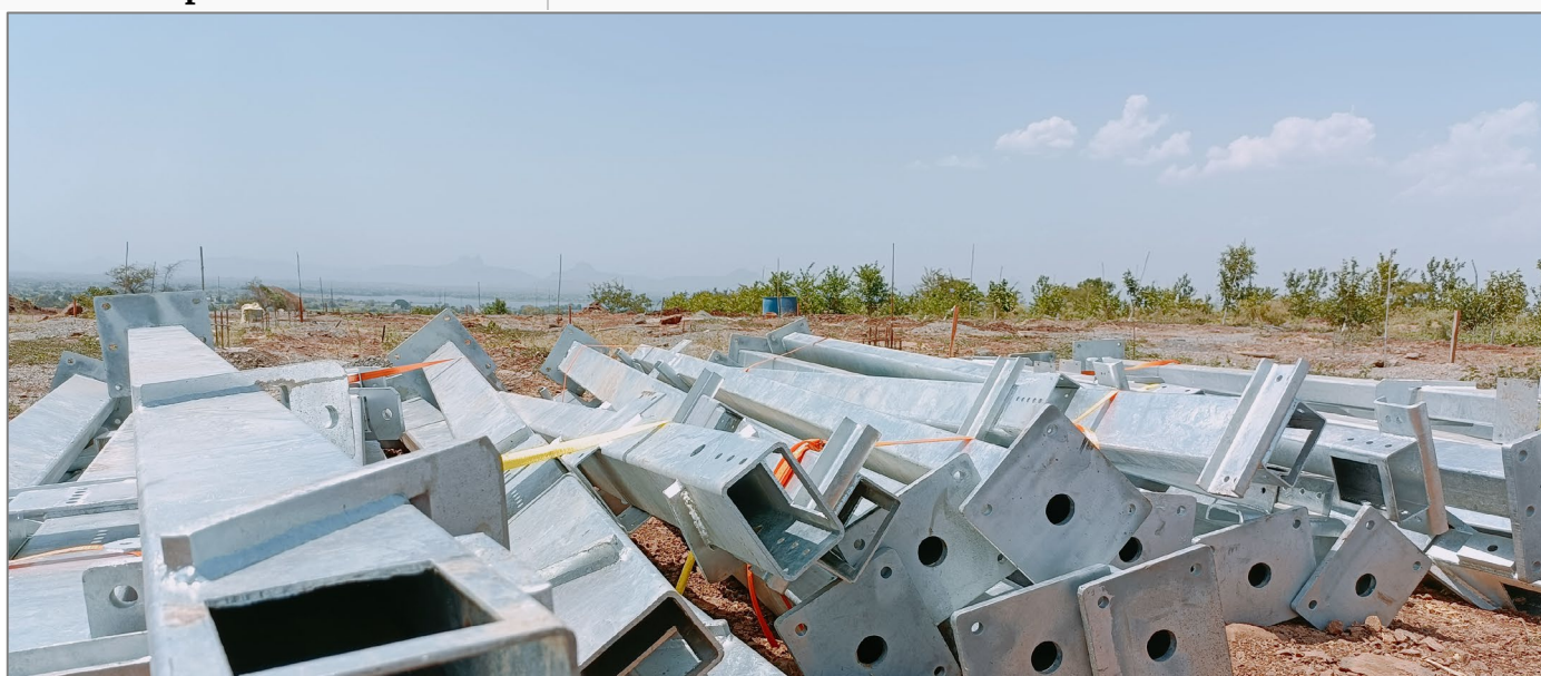
Figure 54: In the front, columns that will soon be mounted during the construction of the agrivoltaics plant near Nashik (Credit: GIZ)
