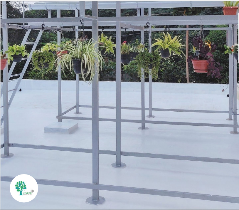
Figure 43: Hinren APVRT structure and white heat seal paint (l), generation profile (r) (Credit: Hinren/Enphase)
