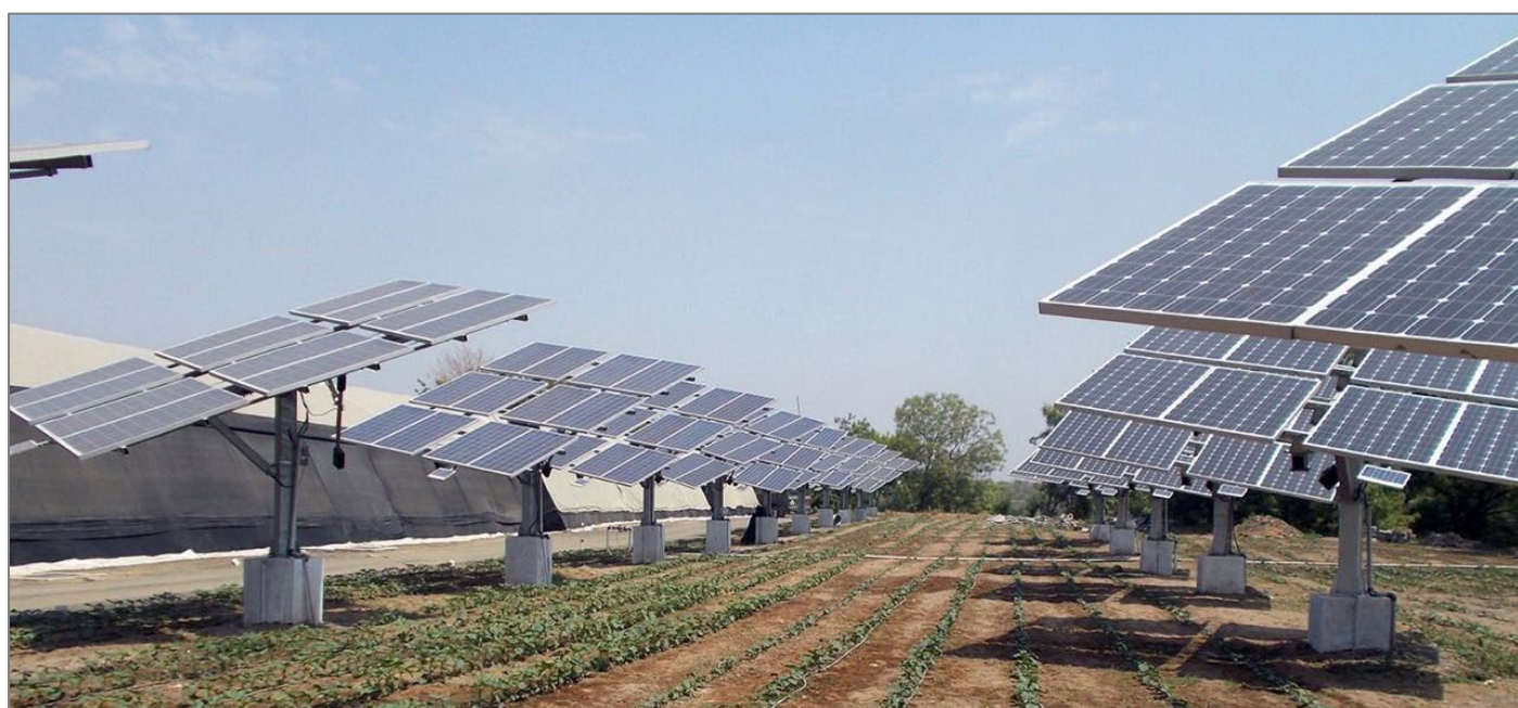
Figure 25: Agrivoltaics with 2-axis tracking and drip irrigation (Credit: Jain Irrigation)
